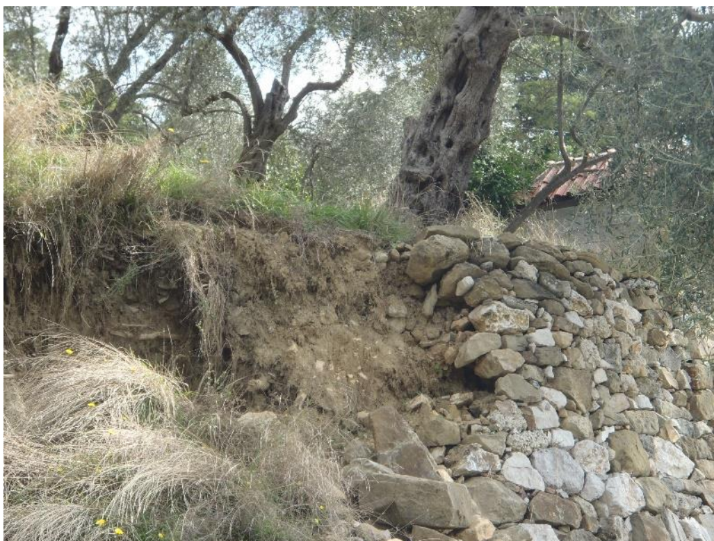
Figure 8: Terrace wall damaged in Prezë
