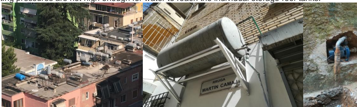
Customer storage tanks in Tirana and booster pump connected directly to UKT network
