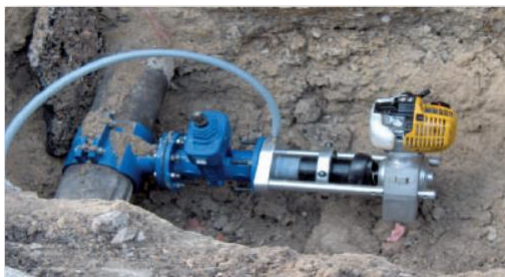
Under pressure drilling to DN-50-200 (source: E.I.E. website)
