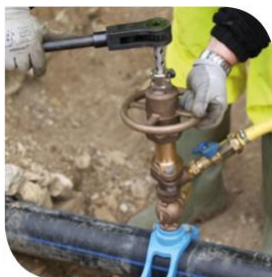
Under pressure drilling To DN 20-40 (source: Sainte-Lizaigne website)
