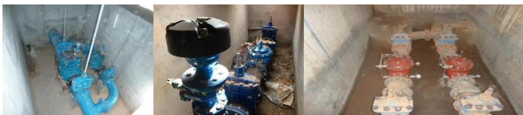
Example of PRVs installed at the inlet of DMAs to regulate the inlet pressure to the area
