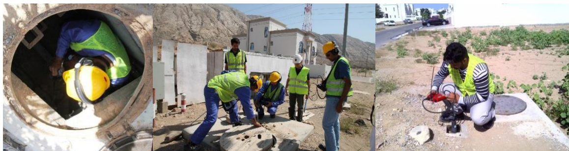
Example of leakage teams working on site using electroacoustic detection and correlation
